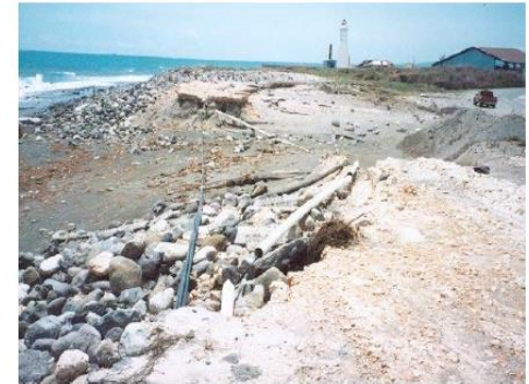
Figure 9: Hurricane Ivan's Disruption of Shoreline at Eastern End of Runway, NMIA Source: Cowill Lyn, NEPA, Jamaica
