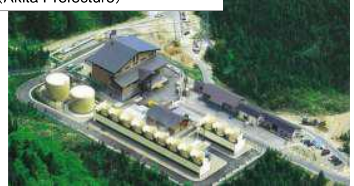
Uenotai Geothermal Plant (Akita Prefecture)
