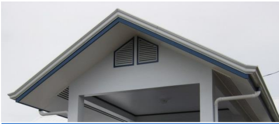
Roof and Soffit Vents
