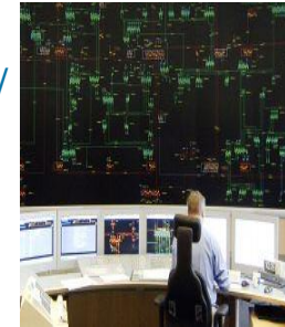
Source: Amprion GmbH
