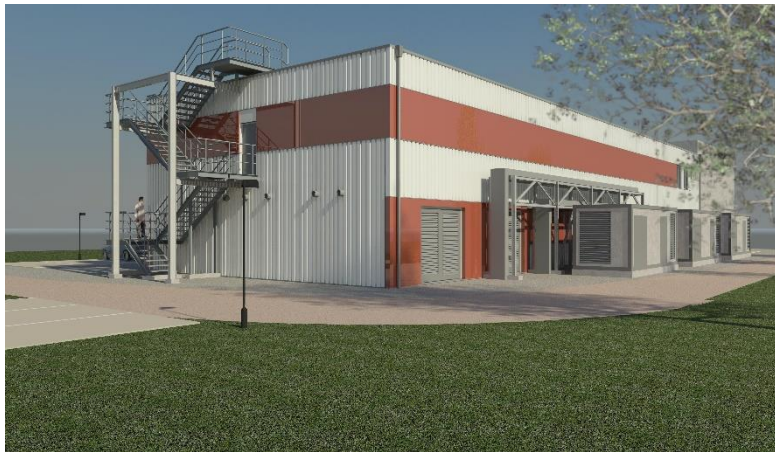
Aachen: 5 MW hybrid facility with li-ion and lead-acid
