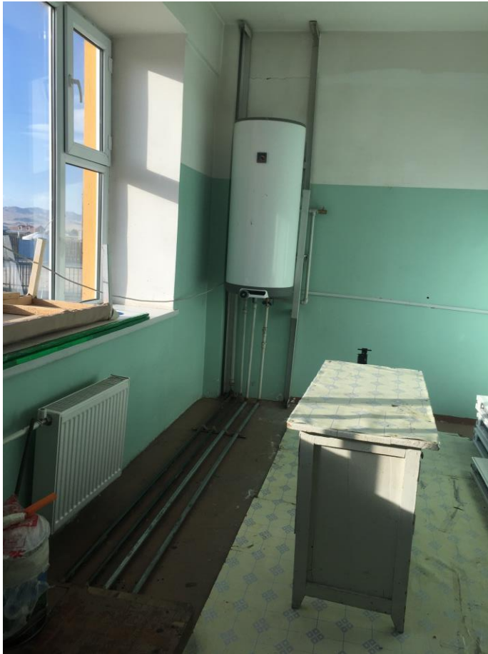
System control room before
