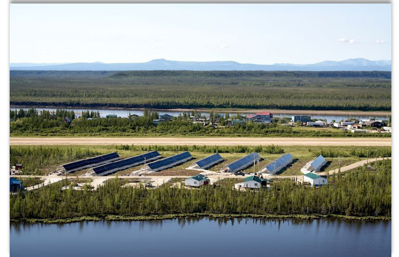
SREE VYAH OLD CROW SOLAR PROJECT Photo credit: GBP Creative
