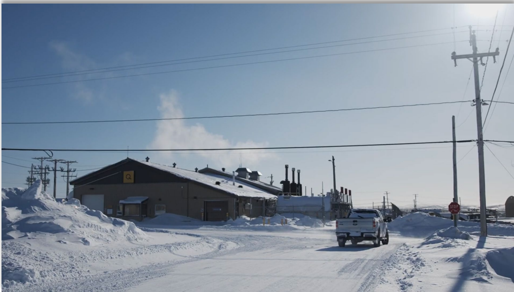
Diesel generating station in KUUJJUARAAPIK, Nunavik, Québec
