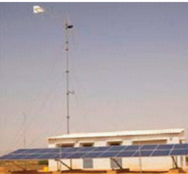
Image 5: Sine Moussa Solar Wind Diesel Hybrid Power Plant © www.peracod.sn
