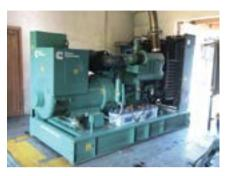
oil and imported diesel fuel. Coconut oil blends of up to 50% were successfully trialed. After the trials, the engine was stripped and inspected and it was confirmed that there was no damage resulting from the use of coconut oil as a fuel source.
