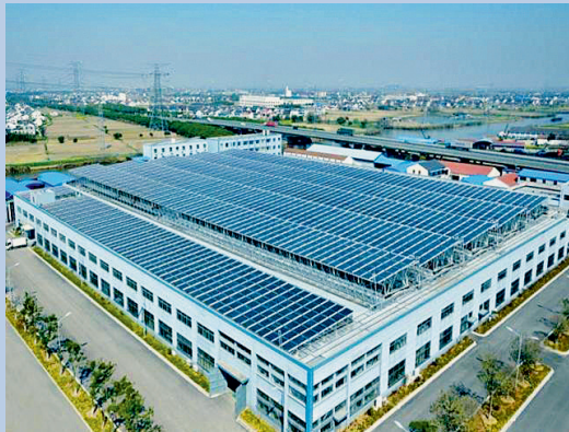
Figure 8: Installation of 7 460 m 2 of ETC in a printing and dyeing plant in China
