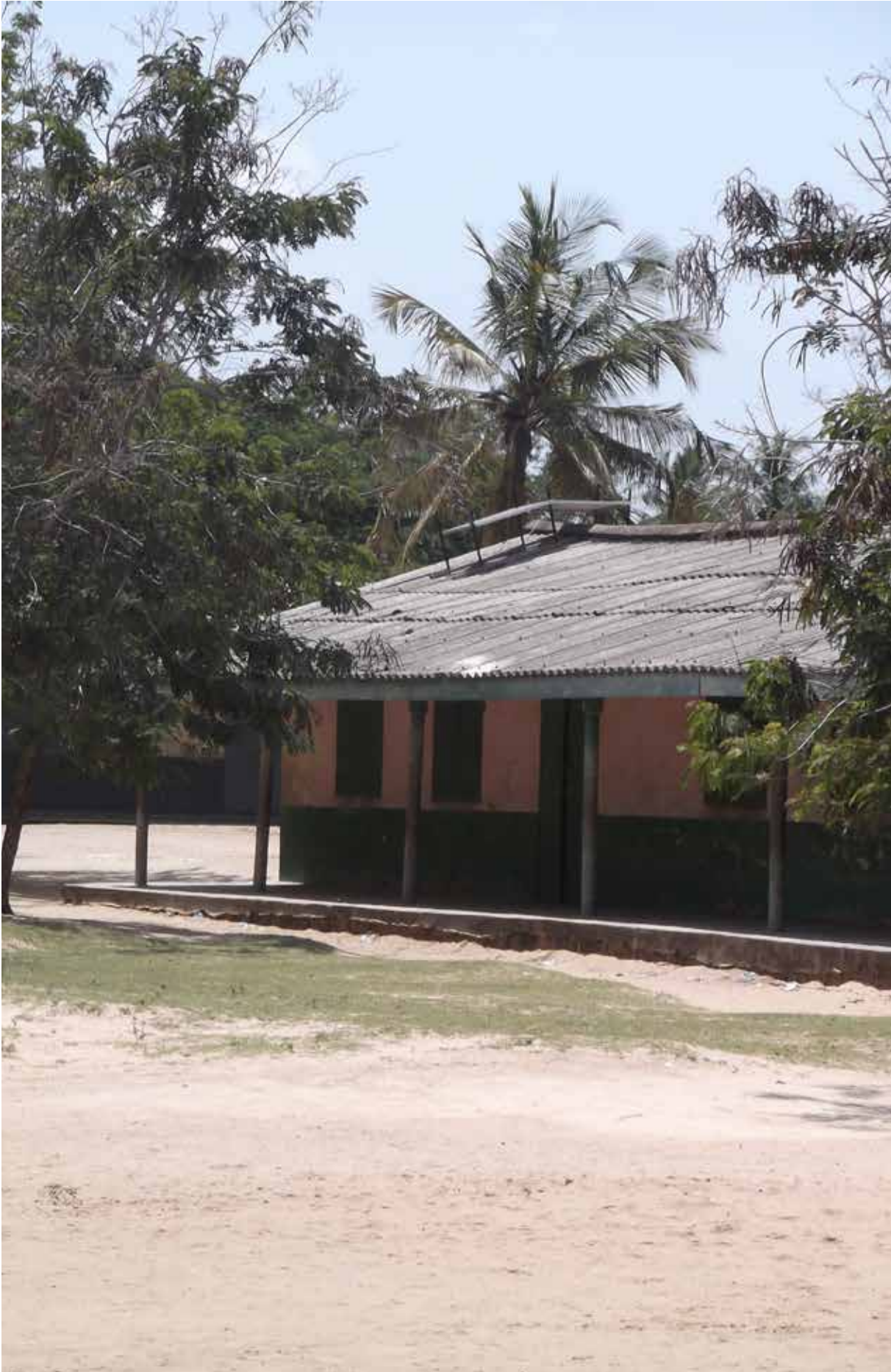
Solar PV for a school in island community
