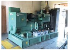
of up to 50% were successfully trialed. After the trials, the engine was stripped and inspected and it was confirmed that there was no damage resulting from the use of coconut oil as a fuel source.
