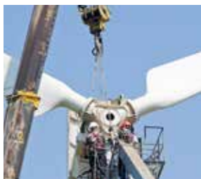
Dismantling the project
