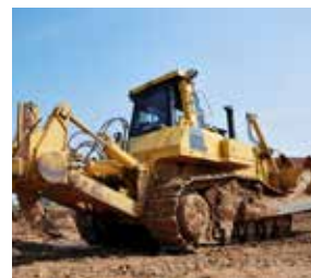
Clearing the site
