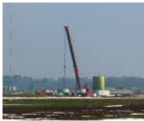
Site preparation and civil works
