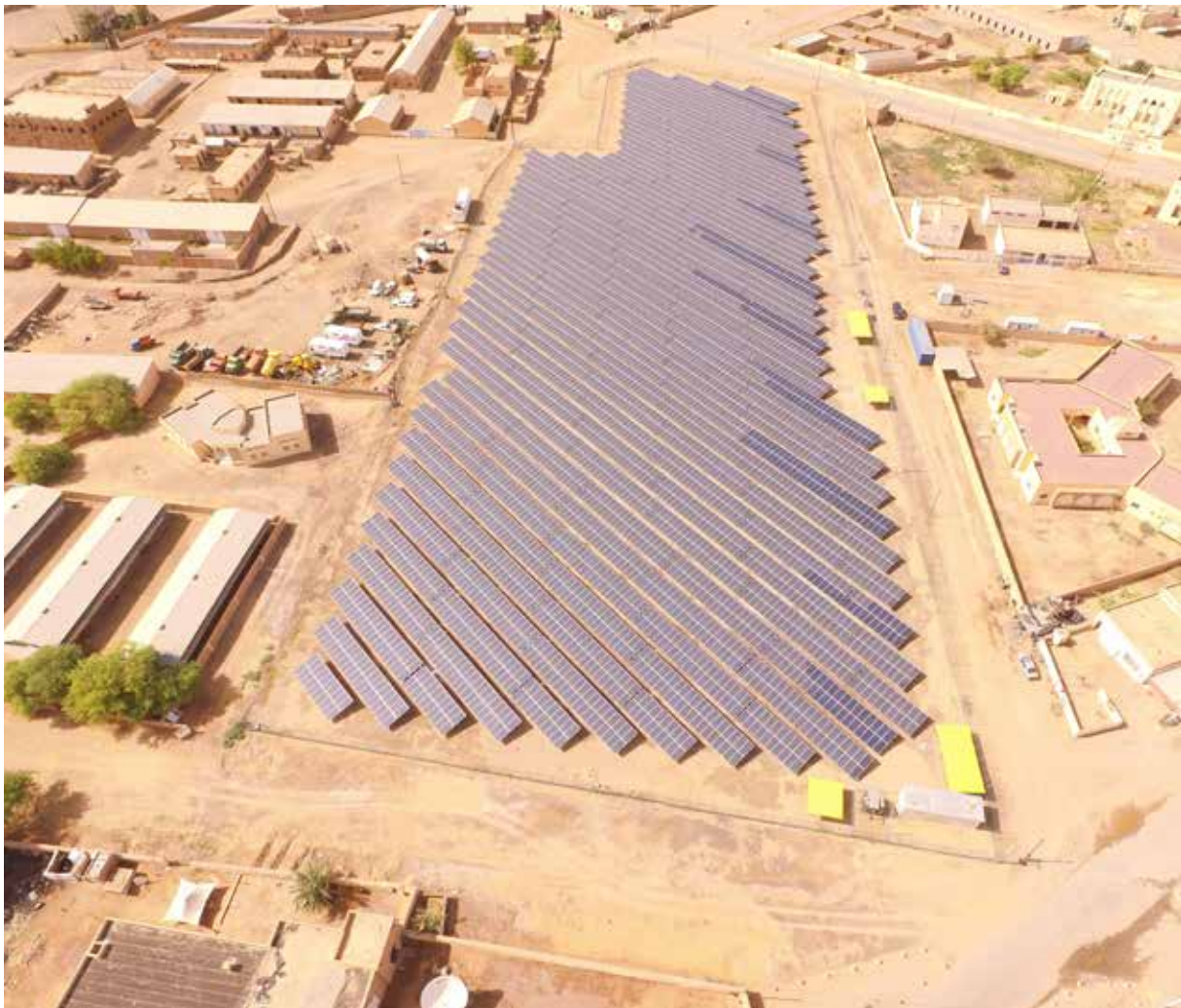
16.6 MW solar PV facility for Mauritania's Rural Electrification Programme
