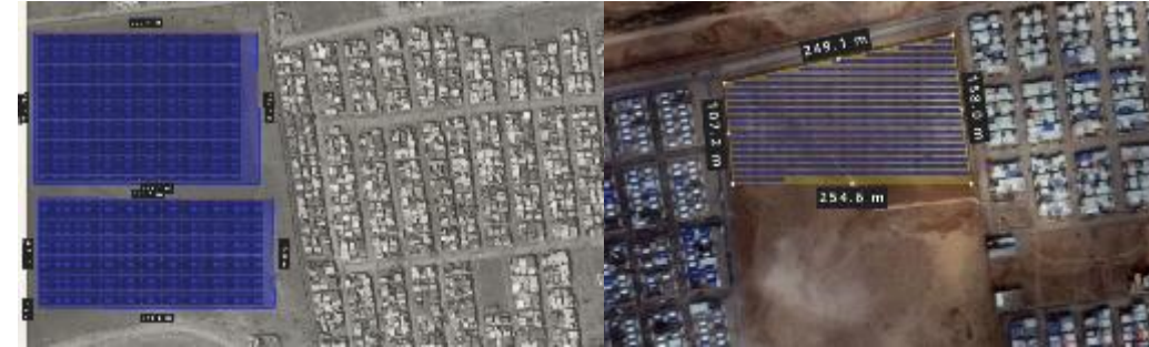
6.6 MW solar PV installation in Domiz 1 (left) and a 2.5 MW solar PV installation in Domiz 2 (right)
